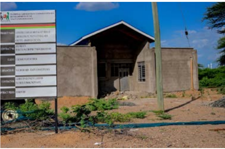
The Digital Hub constructed by the Tiaty Constituency NG-CDF. The project is in the final stages of completion.
